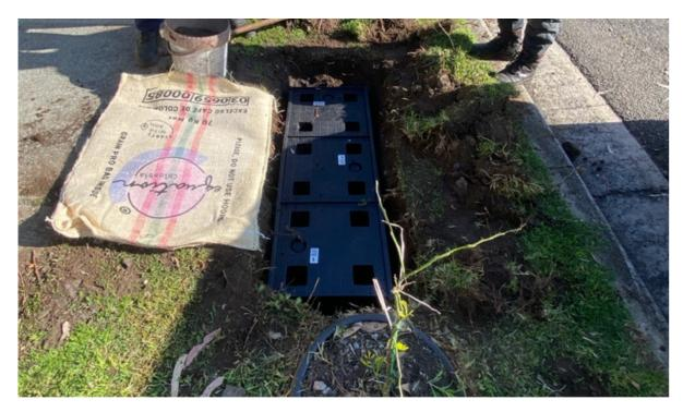
· L to R: Coffee beans hessian sack, Waterups wicking cells in channel in trench, struggling fruit tree in the foreground - the trench and wicking cells lead to the edge of the tree roots and rain drains from the path and verge downhill to the tree roots
